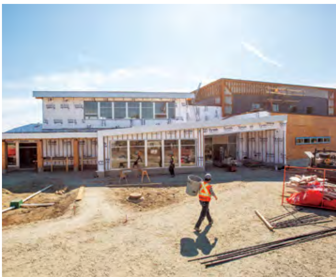
Below: A work site at Snuneymuxw First Nation.
